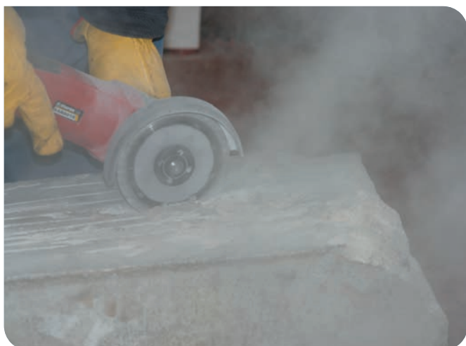
CUTTING WITHOUT AIR SUCTION PROTECTION GUARD.
